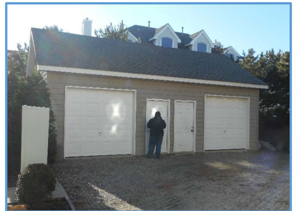
30' x 20' Storage Shed (Between Townhomes 300 & 400)
