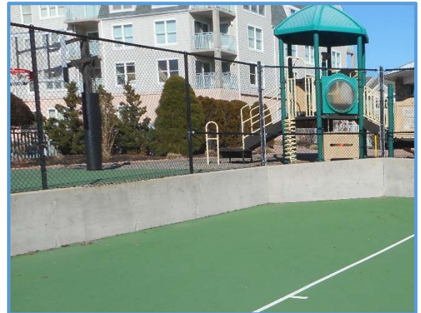
Poured Concrete Retaining Wall
