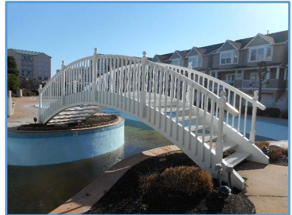
Wooden Pedestrian Bridge (Centre Court Pool Area)
