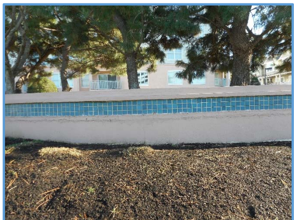
Masonry Concrete Retaining Wall
