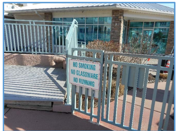
4' Aluminum Fence (Centre Court)
