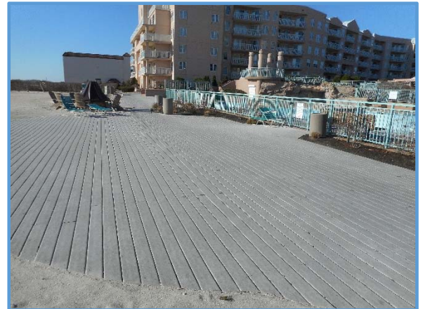
Composite Decking (Ocean Side)
