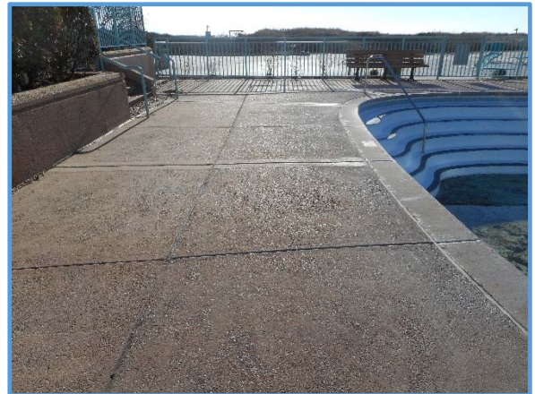
Concrete Pool Deck (Ocean Side Pool Area)
