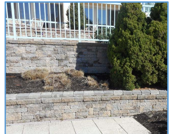
Concrete Field Stone Retaining Wall
