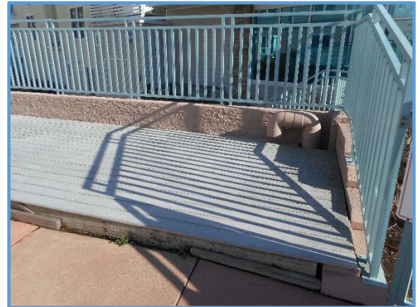
Composite Decking (Centre Court)
